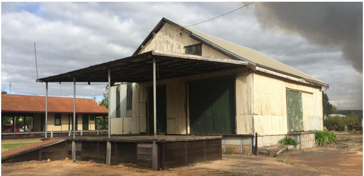
Figure 1: Original Donnybrook Packing Shed before restoration and adaptive reuse
