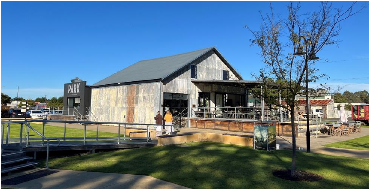
Figure 2: Donnybrook Packing Shed after restoration and adaptive reuse (external)
