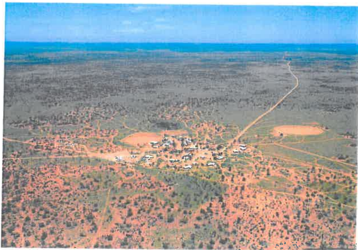
Tjuntjuntjara from the air.
