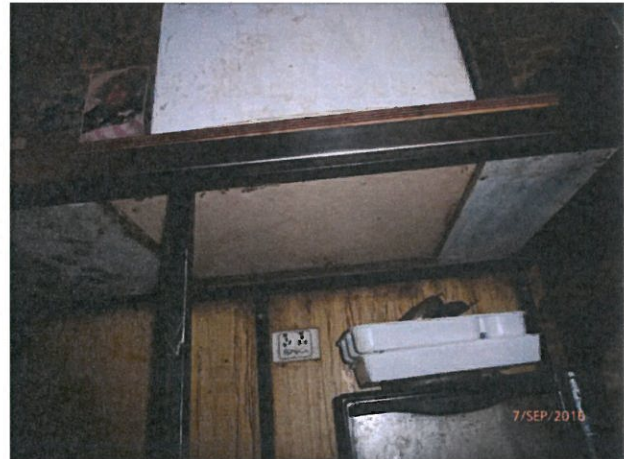
House 9 – As previous
